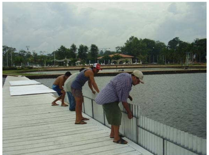
Installing dam boards
